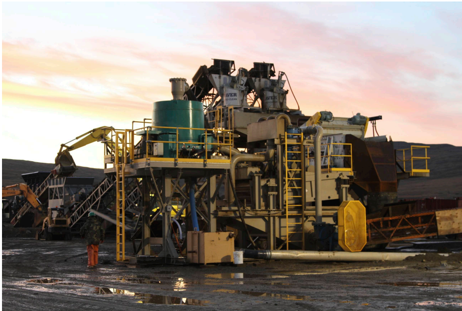
Phase 2 Plant in 2011
